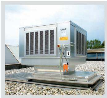
Colt Coolstream can be combined with Coltair Inflow Units to provide highly efficient evaporative cooling, thereby reducing running costs.
