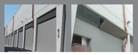
Side vents fitted externally with Colt Universal Louvre in line with surrounding Colt Louvre panels.
