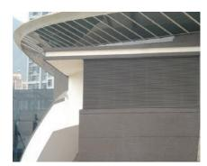
Universal Louvre for plant room ventilation and for controllable air inlet for the smoke extraction system.
