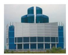
Triple bank facetted circular louvre installed to handle the high air volumes required and to provide maximum rain protection even in typhoon conditions.
