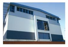
ERD louvre panels on the plant room, and Solarfin solar shading panels.
