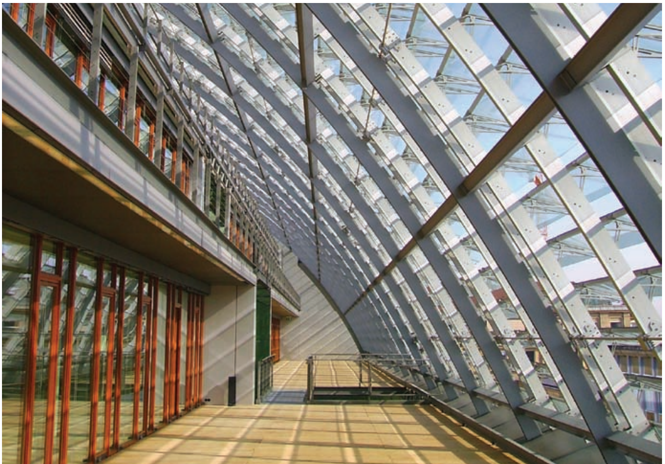
Koeningsbau Passagen, Stuttgart, Germany - A transparent movable glass roof reveals the sky to shoppers, as sophisticated technology provides shelter from the direct influence of the elements.
