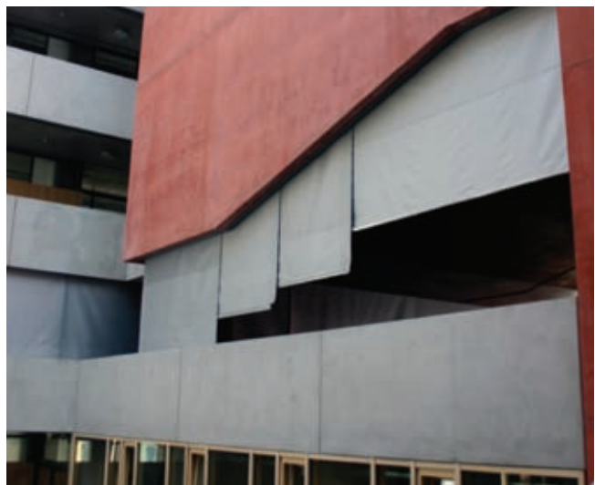
FH Frankfurt – smoke curtains prevent smoke moving from one zone to another
