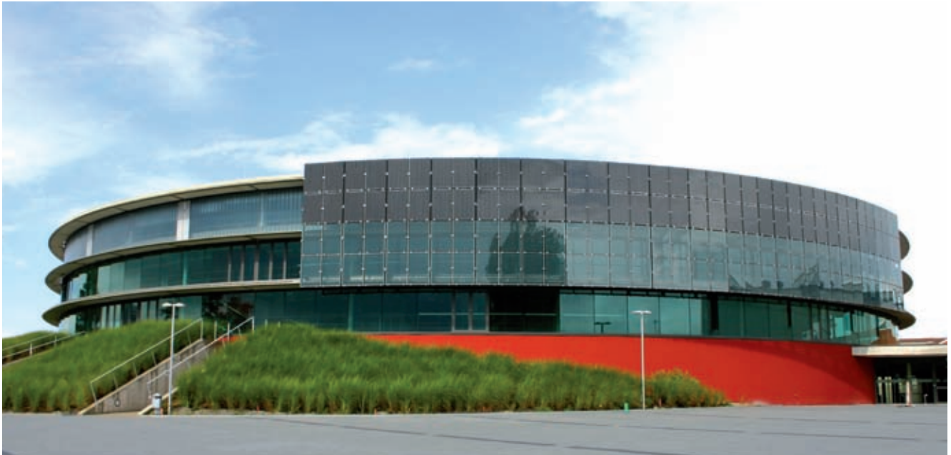
EWE Arena, Oldenburg, Germany - Colt designed and supplied a movable solar wall complete with photovoltaic cells to provide both solar shading and the generation of electricity
