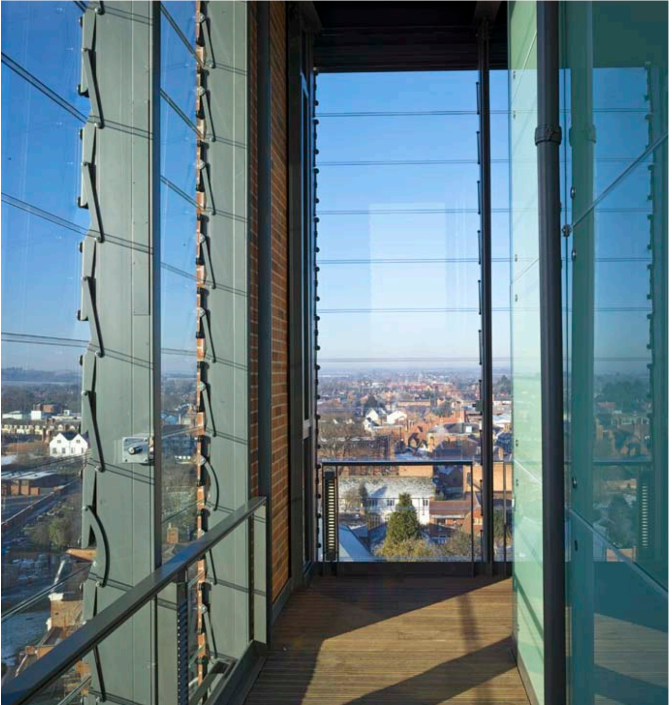
Royal Shakespeare Company, Stratford, UK - 4-sided movable LS-4 glass louvred ventilator
