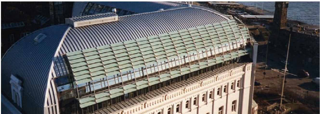
Hotel Hafen, Hamburg - Fritted glass louvre system, enabling daylight to enter the building through the roof whilst reducing solar heat gain
