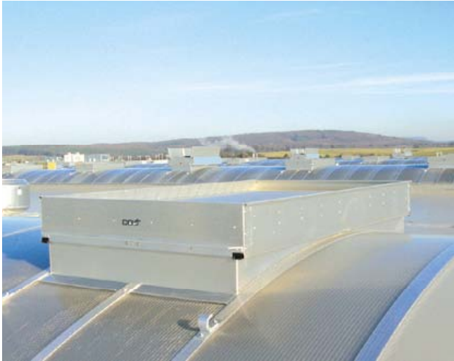
Colt polycarbonate barrel vault systems are highly insulated and allow the integration of ventilation and shading elements
