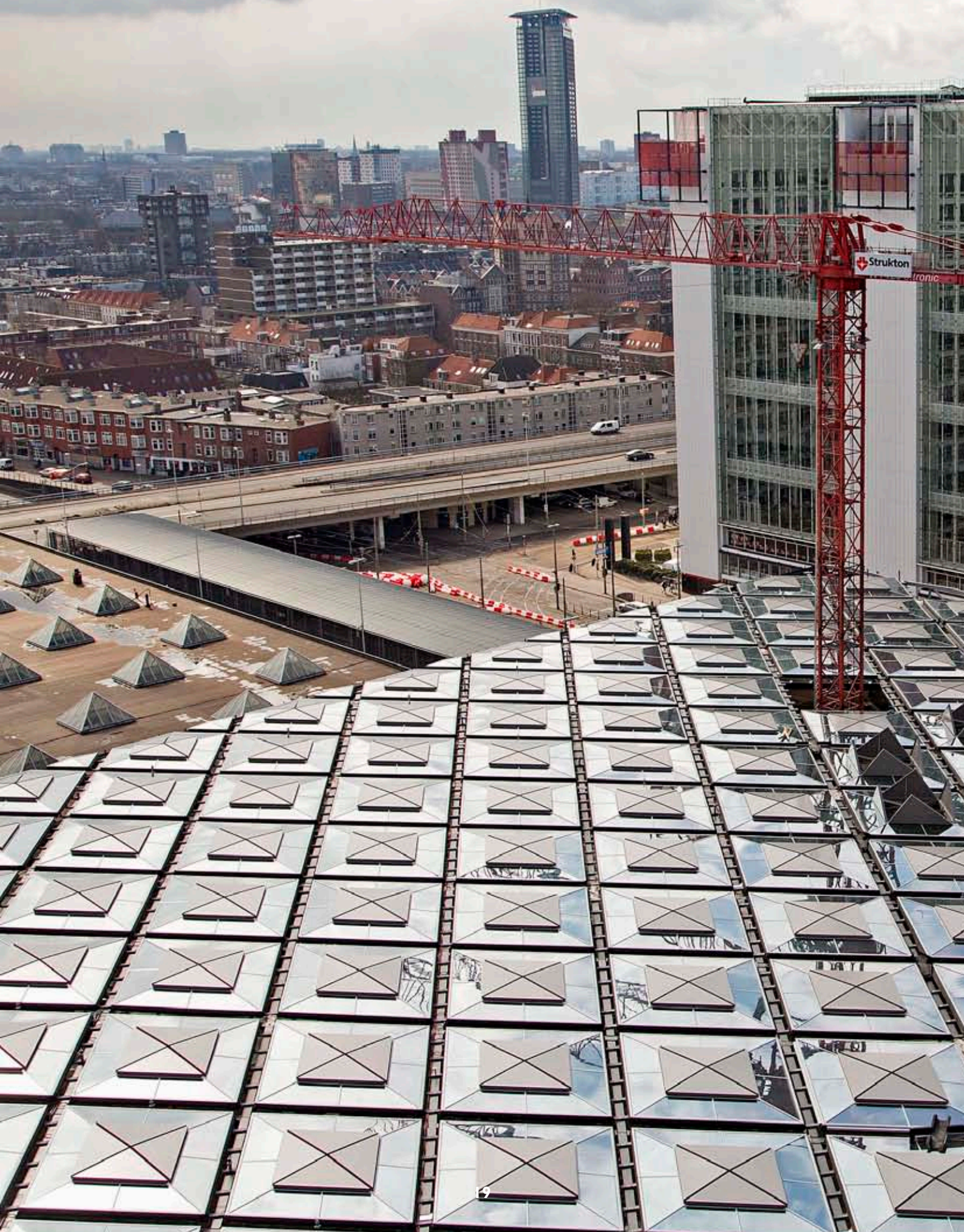
OVT railway terminal, The Hague - Colt provided the complete glass roof including Firelight natural ventilators and all associated framework
