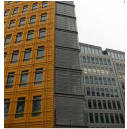
Central St Giles, London - movable glass louvred ventilator
