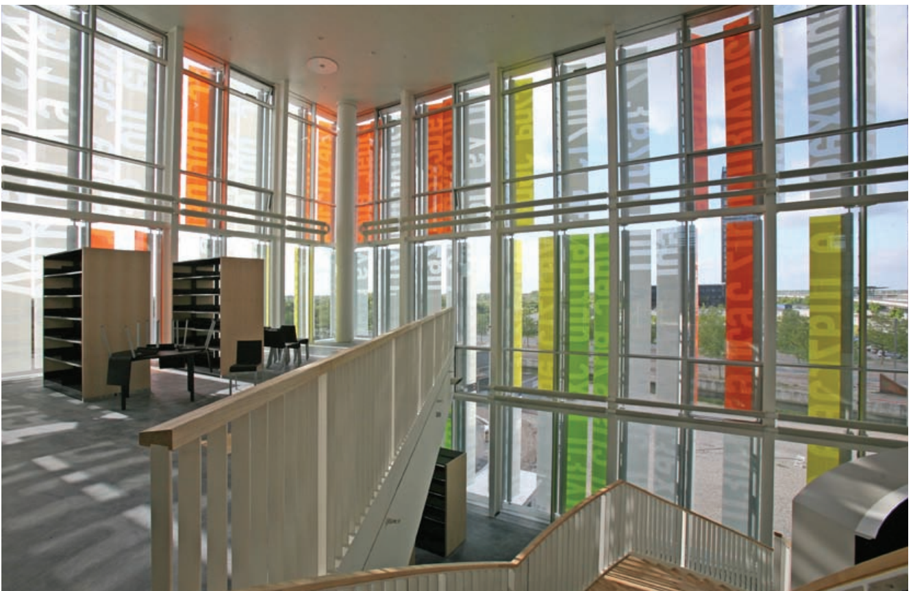
Ørestandens Gymnasium, Copenhagen, Denmark. - Colt designed and installed 700 laminated and printed bespoke Shadoglass glass louvres over an area of 1700m 2 of façade for shading and ventilation. The different colours, films and frits provide a youthful and playful appearance.
